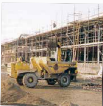
Construction gets underway
